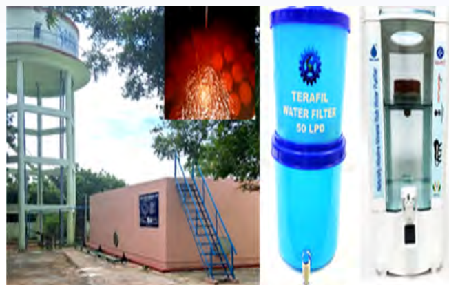
Community size TERAFIL Water Purification Unit (60,000 liters/day)
