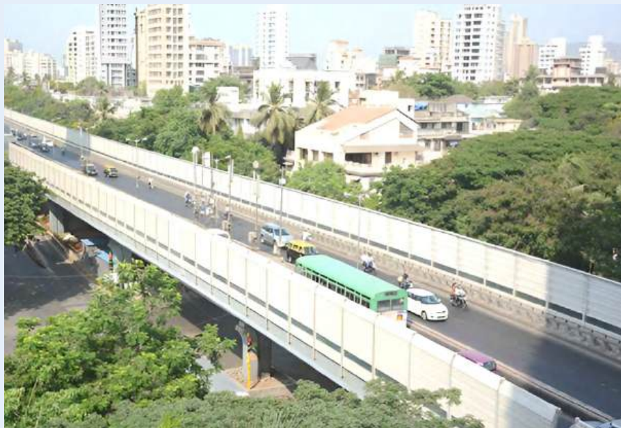
Frequency based noise barrier installed along an elevated urban corridor.
