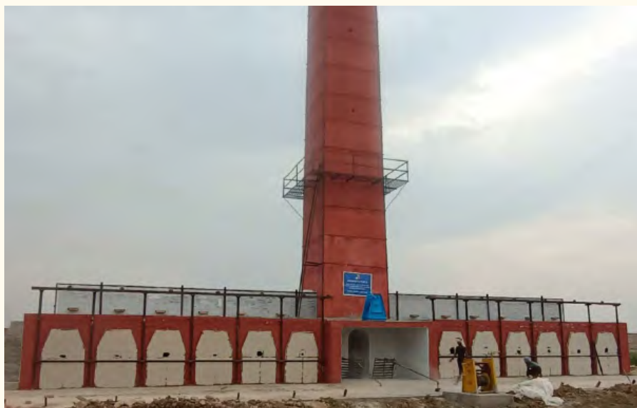
Soft Coke Plant showing Chimney, Winch and Drag Rod
